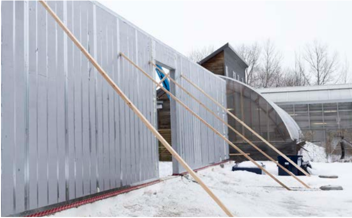
Install temporary wall bracing at MAX 10' intervals during wall panel erection.
