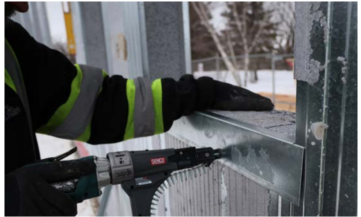
Install a continuous piece of LBC on the bottom of window openings on the interior & exterior panel faces of the opening with edge continuing to jack stud as shown in the photo above.
