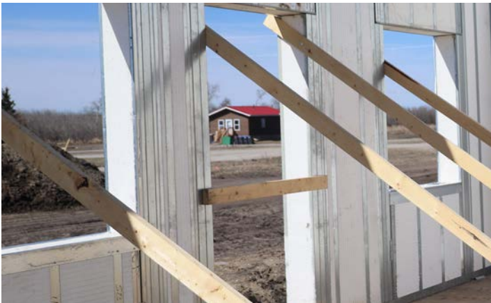
Use the side of rough openings to secure bracing when available.
