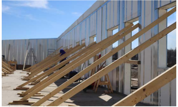
Bracing can be installed to the inside or outside of the building.
