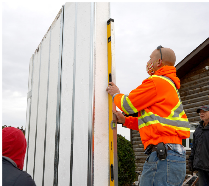
You should have a straight and plumb starting point.
