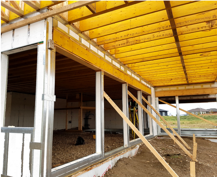
Install temporary wall bracing at MAX 10' intervals during wall panel erection.
