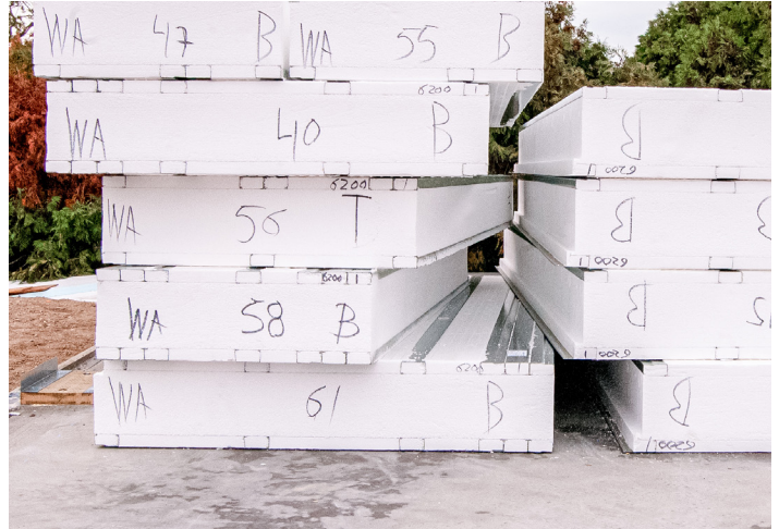
The provided Installation Drawings show an element number for each panel in the floor plan, which appears on the top and bottom end of each panel.
