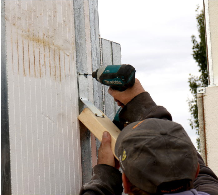
Use appropriate screws to fasten bracing.
