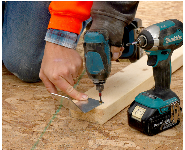
Field Bent Connector Plate can be used as temporary brace connectors.
