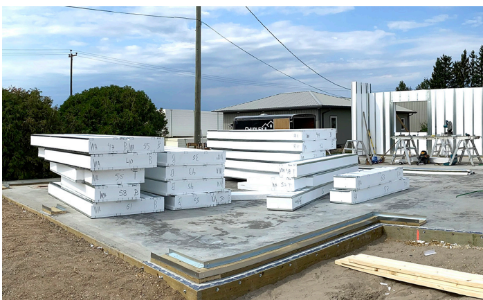
When unloading, stack the panel bundles where they can easily be accessed for distribution once the base track is installed.
