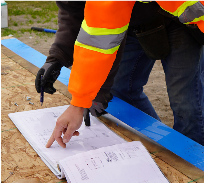
Determine sequence of panel assembly. It can initiate in any building corner, with the direction of assembly as shown on your installation drawings.
