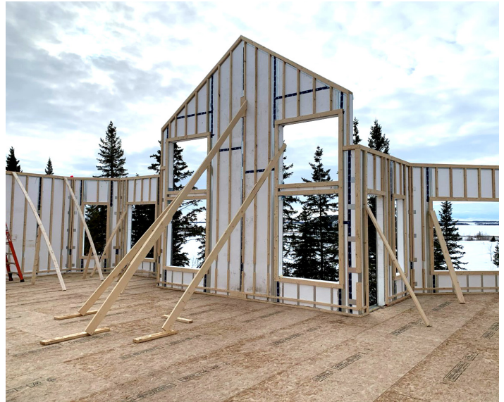
Bracing can be installed to the inside or outside of the building.
