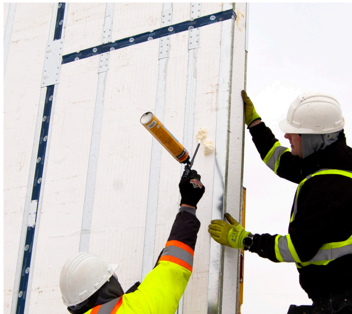
Apply foam (in a corner butt joint application) between the panels from top to bottom, and push panels together.
