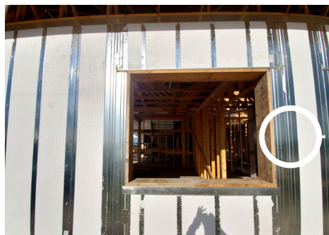
Take exterior photos showing 15-20 foot sections of wall per photo.
