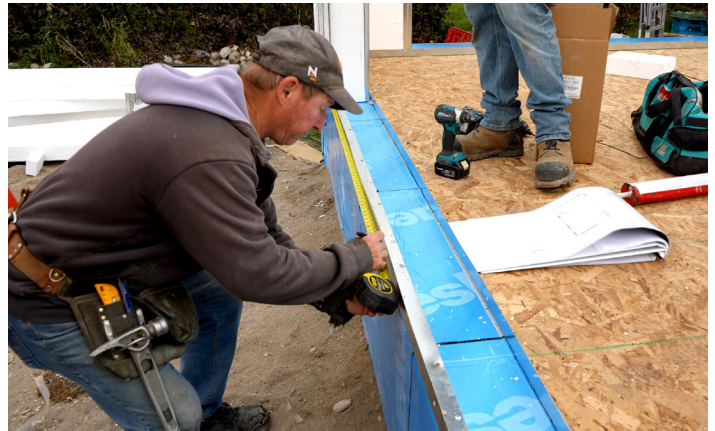
Identify opening starts and stops and mark for reference. You will adjust the panels to these during installation by leaving slight gaps between panels on the interior wall.
