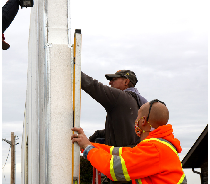
Ensure walls are straight as you brace to minimize adjustments.
