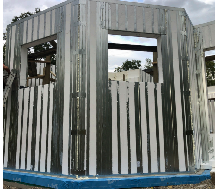
Insulated Header panels are built 3/8" shorter than the opening to allow for placement and foaming.
