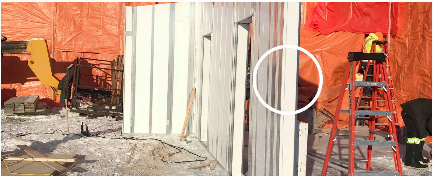
The leading edge of a ship lap panel always points the intended direction of assembly.
