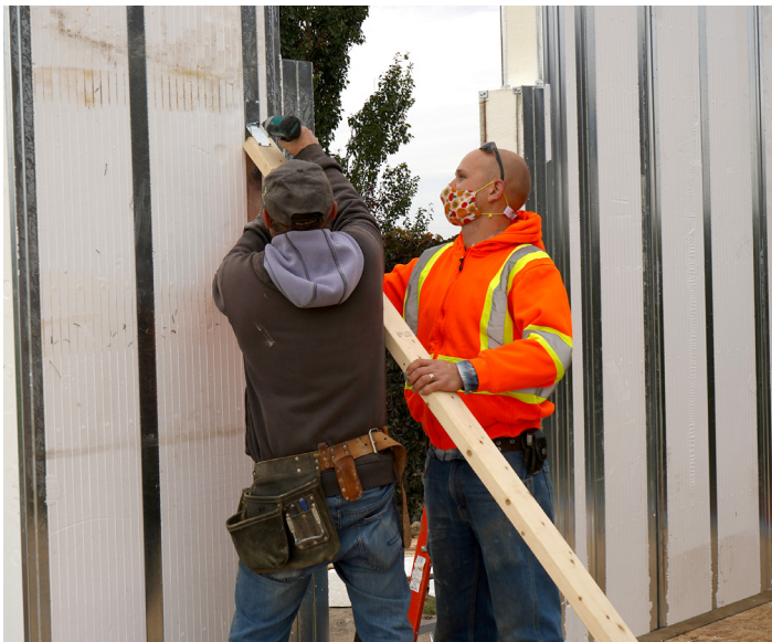
Use the side of rough openings to secure bracing when available.
