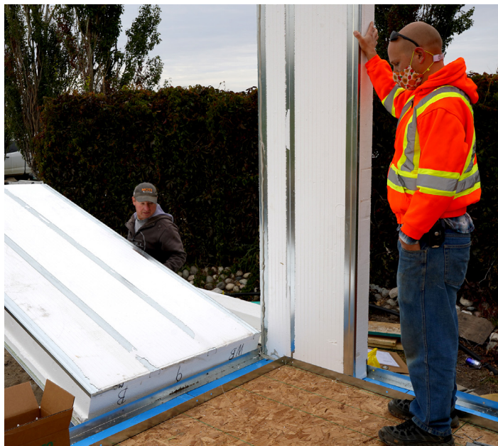
Place other corner panel approximately 1" from the first panel.
