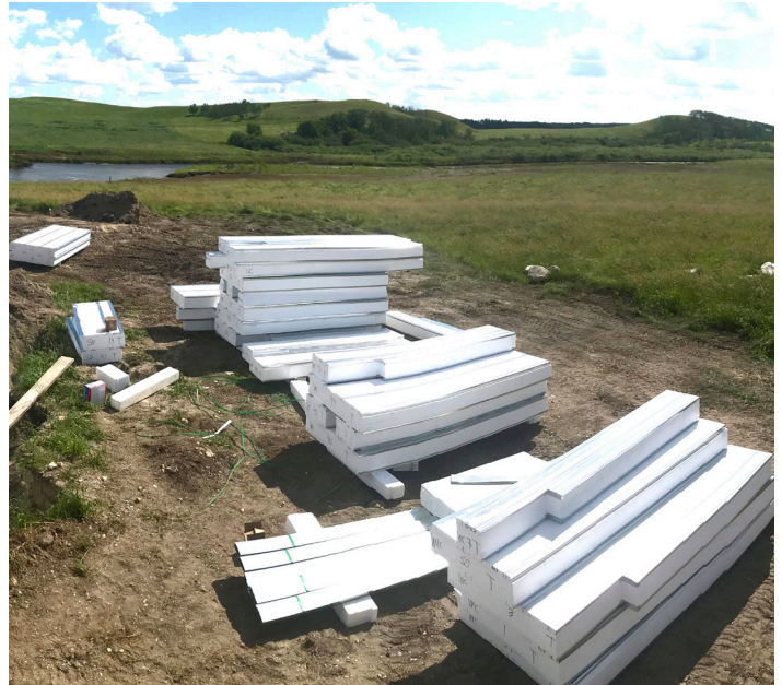
Unbundle and lay the panels near their install location for easy access during erection.
